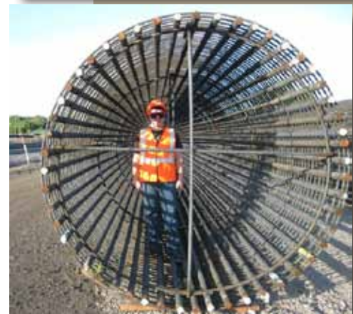
Ryan Hoensheid standing inside one of the reinforcement cages for an overpass bridge in Salt Lake City, Utah.
